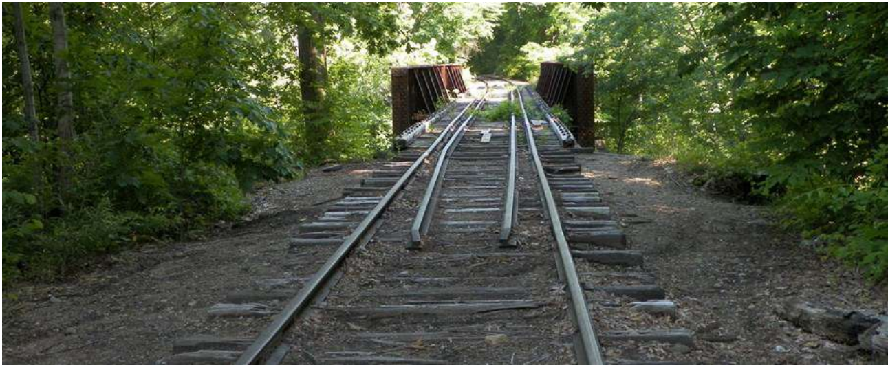
Figure 4.5 Valley Railroad State Park: Deteriorating track and vegetation on Higganum Cove bridge
