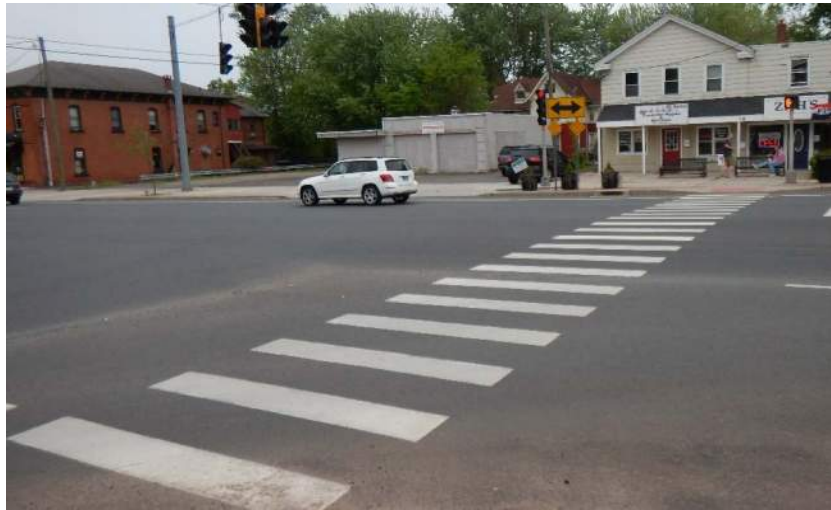
Crosswalk at the intersection of Route 66 and Route 17A (Main Street)
