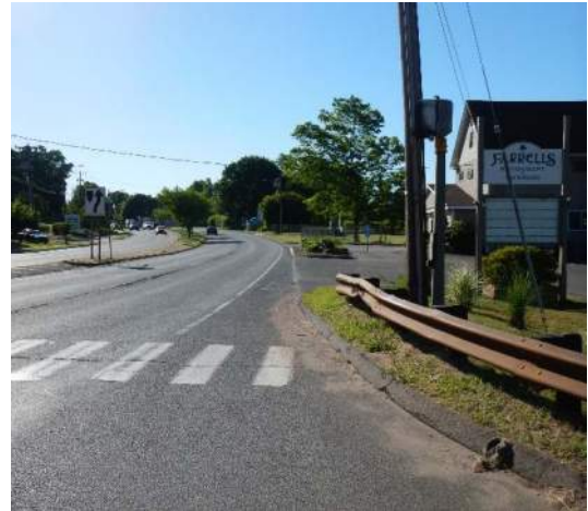
Non-compliant ADA pedestrian accommodations at the intersection of Route 66 and Airline Avenue
