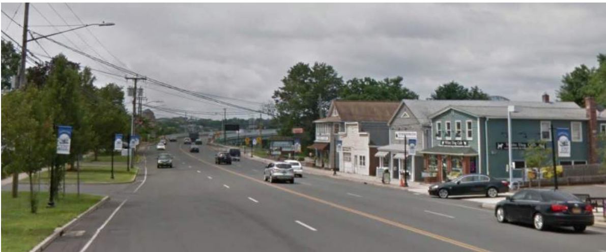
Route 66 in Portland looking West towards the Arrigoni Bridge
