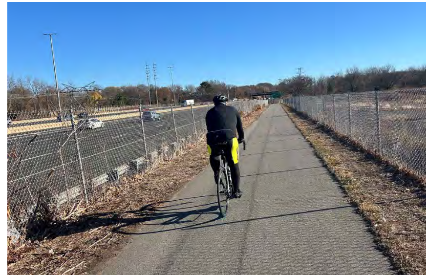
Shared-use path example within an interstate highway ROW (Charter Oak Greenway adjacent to I-84 in East Hartford)
