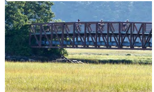
Example trail bridge in Scarborough Maine
