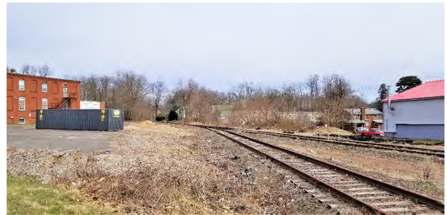
View of the state-owned rail corridor, looking north from Pickering Street
