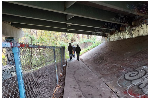
Underpass below Newfield Street looking southwest to Jackson Street
